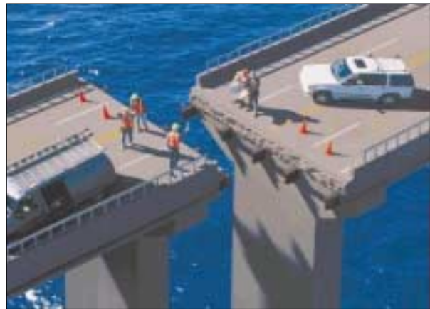
Figure 1. A graphical demonstration of the importance of an accurate and universally accepted spatial geodetic reference network. Left image: The seamless flow of a well constructed freeway that was built with all the construction teams using the same, accurate coordinates. Right image: An imaginary bridge being built with construction teams using different and inaccurate coordinates.
