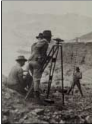
Figure 2. Conventional line-of-sight survey methods that have changed very little from the leveling survey party in the left image ( http://www.photolib.noaa.gov/historic/c&gs/theb1773.htm ), which used a telescopic level similar to the center image ( http://www.surveyhistory.org/index.htm ), to present-day leveling survey parties, which utilize laser levels similar to the Zeiss level in the right image ( http://www.zeiss.com/survey/digital/dini11.shtml ).
