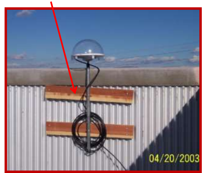
Problem wooden support U-bolts height can change
