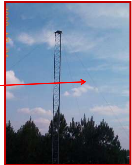
Antennas on towers with guy wires poor stability
